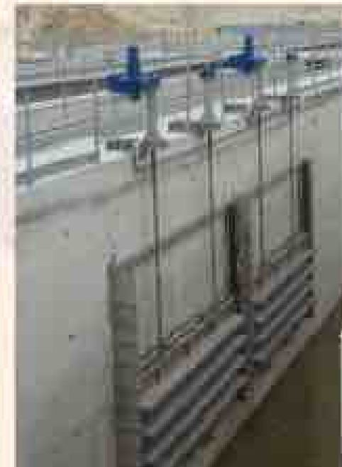
T10 Duplex Penstocks with FOCUS Actuators Series E & ICU Control
