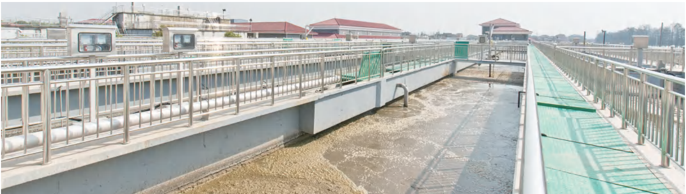
Project Name : The third phase MBR system project at a wastewater treatment plant in Liangzhu, Hangzhou Deploy Time : Year 2015 Model No. : MBR Treatment Capacity : 30,000T/D
