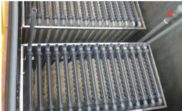
Project Name : An emergency Pump Station Treatment Project in Yuhang District Deploy Time : Year 2018 Model No. : MBR Water Type : Wastewater Treatment Capacity : 5,000T/D
