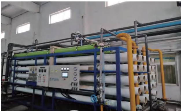
Project Name : Water Resource Utilization and Reuse Project in Shandong Deploy Time : August,2015 Model No. : NF/8040-R85 Water Type : Blending of recycled water, wastewater & RO concentrate Treatment Capacity : 2,000T/D
