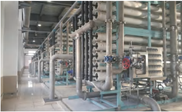
Project Name : Industrial water plant in Dafeng Development Zone Deploy Time : December, 2017 Model No. : LE400FR Water Type : Industrial Wastewater Treatment Capacity : 8,000T/D
