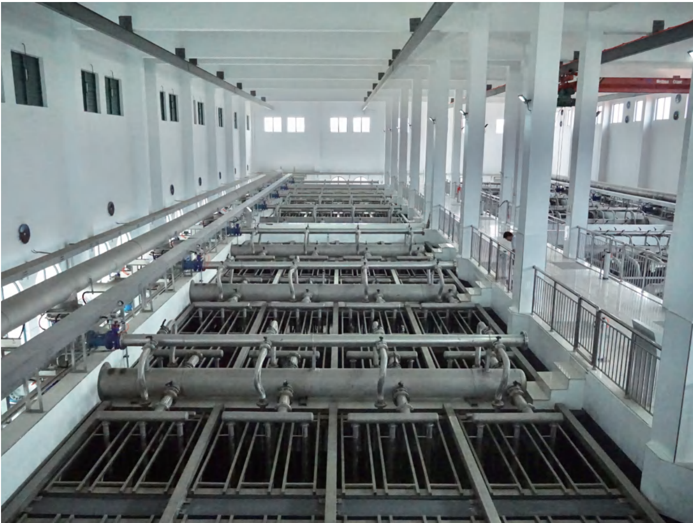
Project Name : A water treatment plant in Yuhang District Deploy Time : Year 2017 Model No. : Submerged UF Membrane - TXP Treatment Capacity : 10,000m 3 /d
