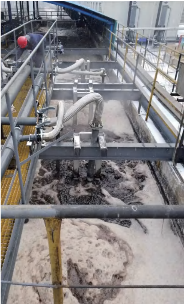
Project Name : Pingshan River Basin Comprehensive Water Environment Improvement Project Deploy Time : Year 2018 Model No. : MBR Water Type : Domestic Sewage Treatment Capacity : 68,000 T/D
