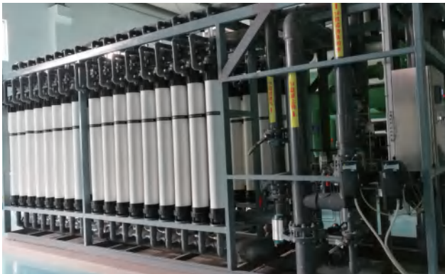
Project Name : A Textile Technology Company in Shaoxing Deploy Time : Year 2019 Model No. : EI-UF-9080-PVDF Water Type : Dyeing and Printing Wastewater Treatment Capacity : 14,000T/D
