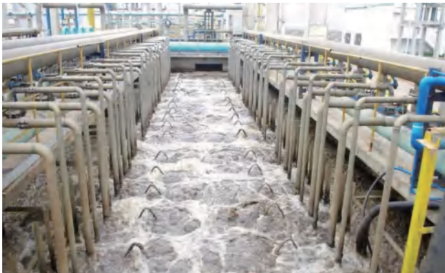
Project Name : Water Purification Project in a Nanping, Fujian Deploy Time : Year 2019 Model No. : MBR Water Type : Domestic Sewage Treatment Capacity : 25,000T/D
