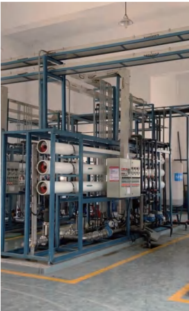
Project Name : A Landfill Project in Zhejiang *Recovery Rate≥85% * COD Removal Rate≥96% *Low treated water color *NF system operation pressure 0.50Mpa *NF system operation temperature:30-39℃ *Permeate Flow : 15t/h
