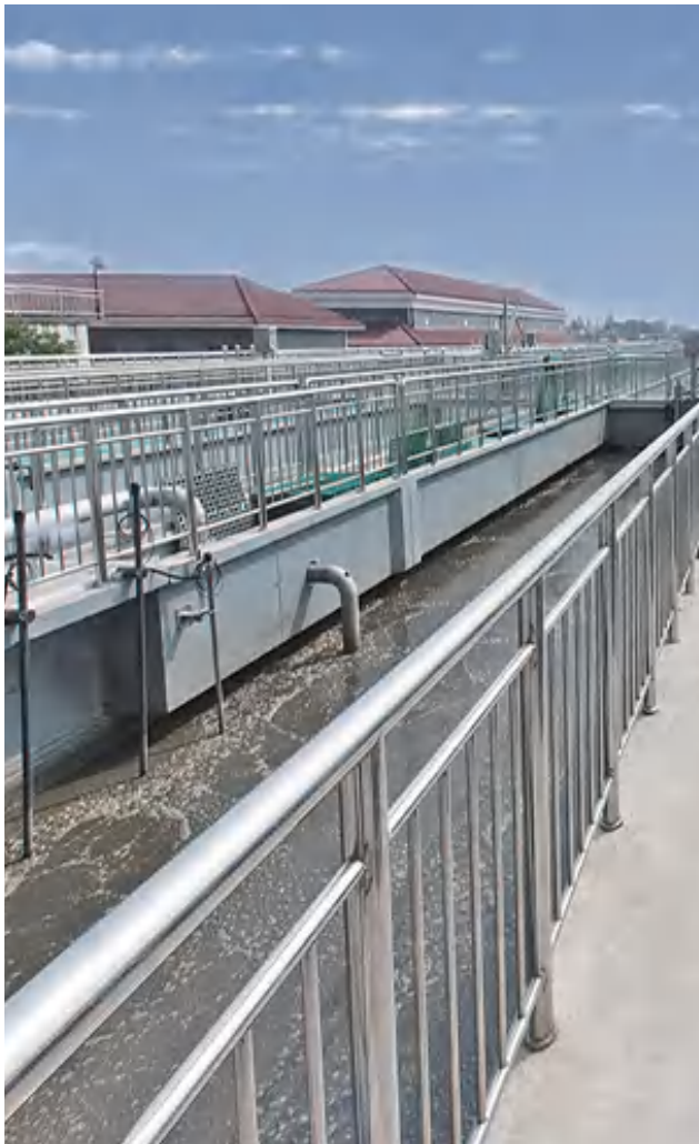
Project Name : A wastewater treatment plant in Chengdu, Sichuan Deploy Time : Year 2017 Model No. : MBR Water Type : Domestic Sewage Treatment Capacity : 10,000 T/D
