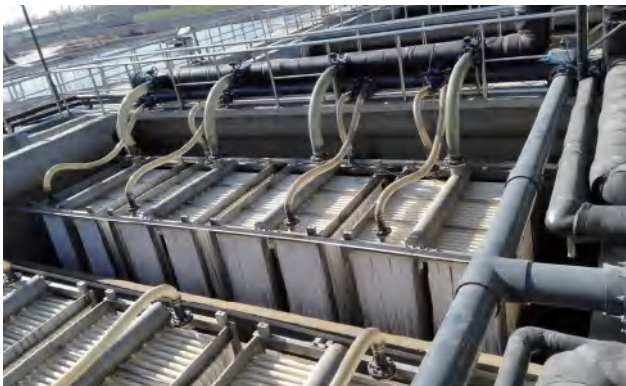
Project Name : A sewage treatment plant in Bozhou District Deploy Time : Year 2019 Model No. : MBR Water Type : Industrial Wastewater Treatment Capacity : 4,000 T/D
