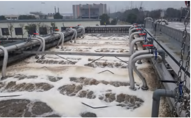
Project Name : Emergency Treatment Design Project in Yixing City Deploy Time : Year 2020 Model No. : MBR Treatment Capacity : 15,000T/D
