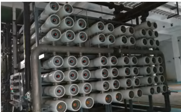
Project Name : A water quality improvement project in Anhui Replace time : March, 2015 Model No. : NF/8040-R85 Water Type : Underground Water Treatment Capacity : 2,300 T/D
