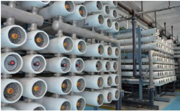
Project Name : A Petrochemical Company in Ningbo Deploy Time : Year 2020 Model No. : BW-400FR Water Type : Industrial Tap Water Treatment Capacity : 21,600T/D
