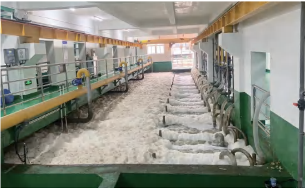
Project Name : Upgrade and Technological Transformation Project of a Electroplating Wastewater Resource Utilization Center Deploy Time : Year 2020 Model No. : MBR Treatment Capacity : 6,500T/D
