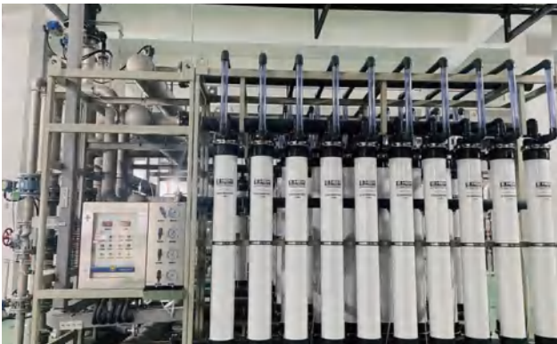
Project Name : A New Energy Technology Company in Hubei Deploy Time : Year 2023 Model No. : EM-UF-8080-PVDF+RO+NF Water Type : Industrial wastewater Treatment Capacity : 300,000 T/Yr
