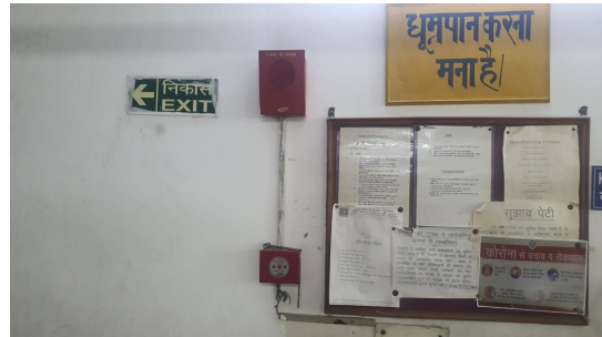
NC - No Instruction for use of Fire Alarm.jpg
