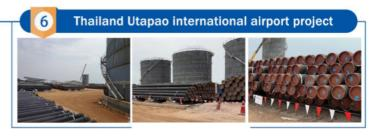
API 5L PSL2 grade BN Internal and external anticorrosion
