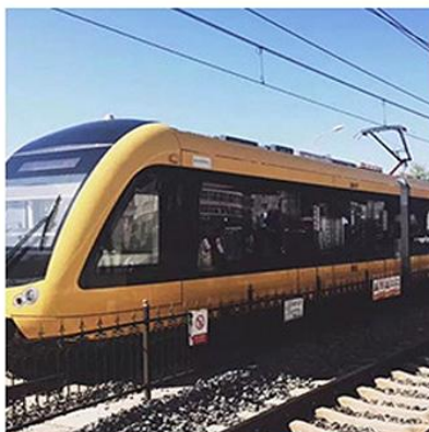
Rail transit equipment
