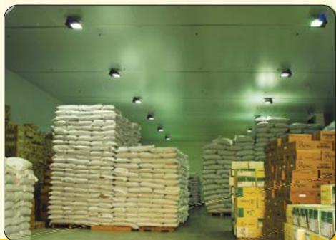
Chiller / Cold Room
