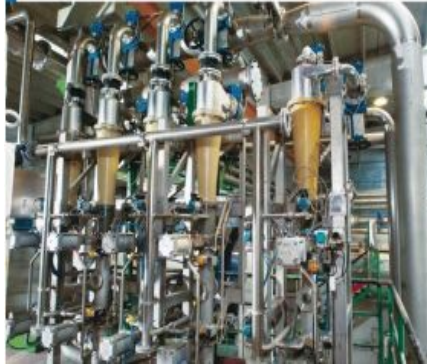
AhiCleaner RB600HD and RB300HD Heavy debris removal at high consistency
